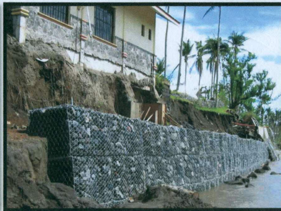
Figure 1. Examples of constructed gabion chekdam
