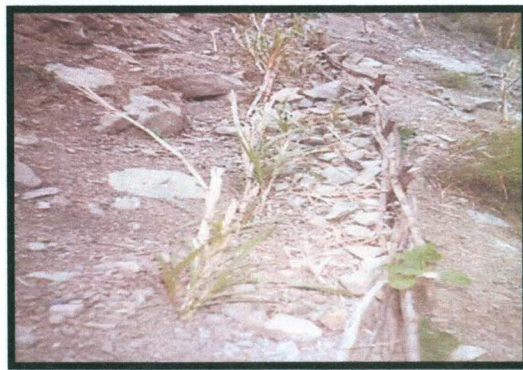
Figure 5.1 Examples of established modified wattling
