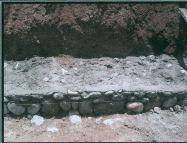
Figure 3. Examples of constructed grouted riprap or stonewalls
