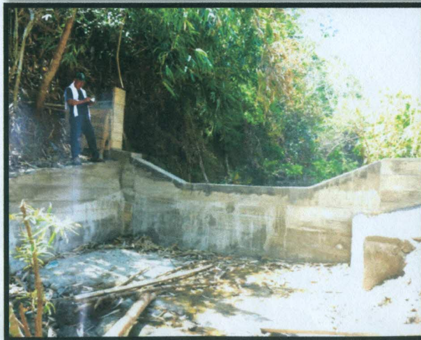
Figure 2. Example of mixed boulder and concrete checkdam
