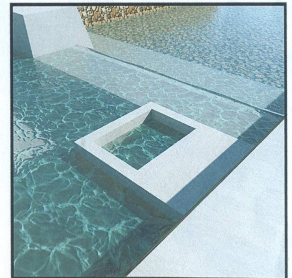
Submersible pump pit
