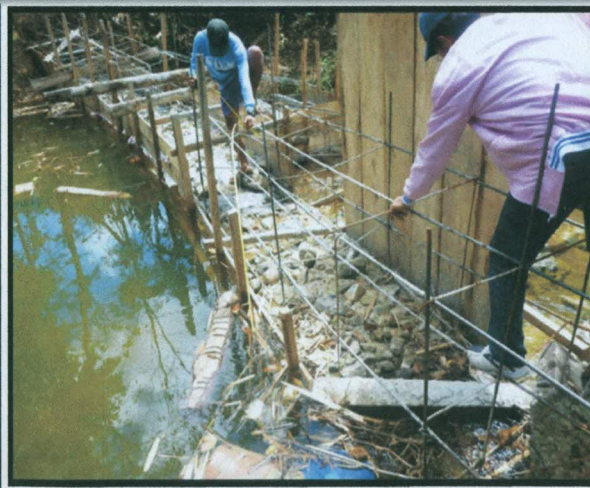
Figure 2. Example of mixed boulder and concrete checkdam
