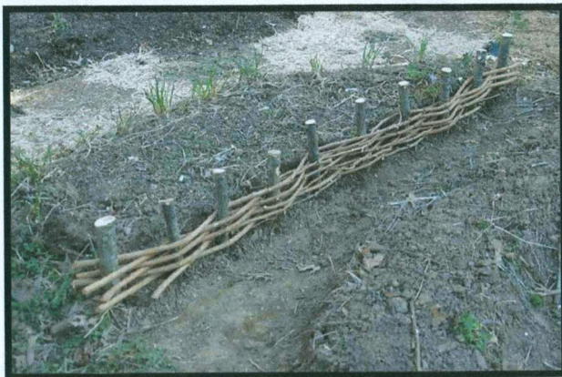
Figure 5. Examples of established wattling
