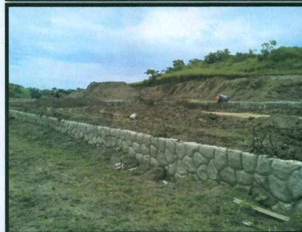
Figure 3. Examples of constructed grouted riprap or stonewalls
